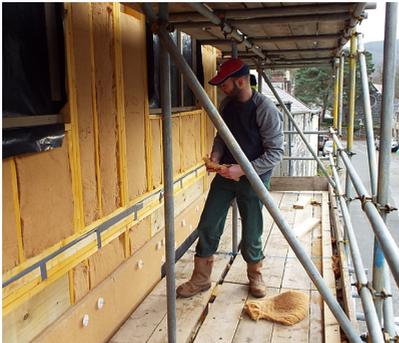
Company Director Gary Newman on site installing plant fibre insulation on a low carbon Williams Homes timber frame housing project
